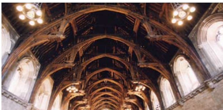
The famous 14th century hammer beam roof at Westminster Hall.
