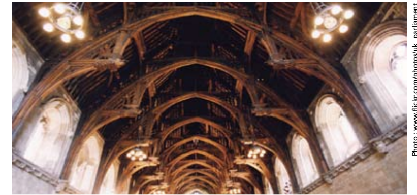
The famous 14th century hammer beam roof at Westminster Hall.
